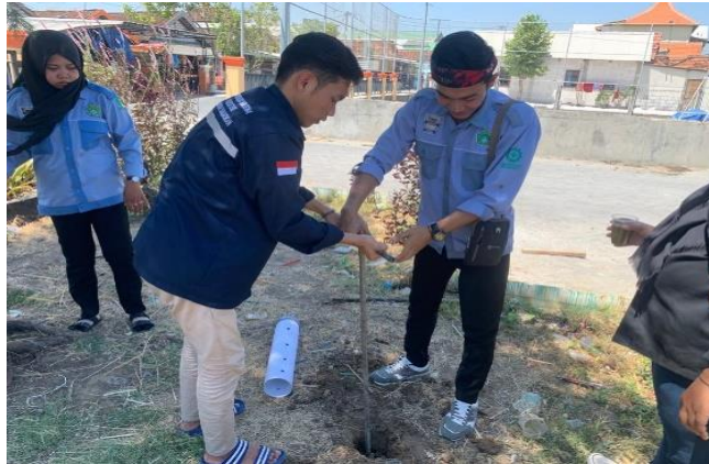
Figure 2. Soil Drilling for Biopore Planting
