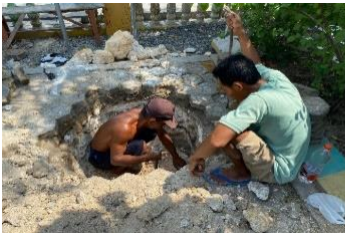
Figure 3. Infiltration Well Digging Process.
